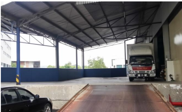
Loading ramp to warehouse entrance 2
