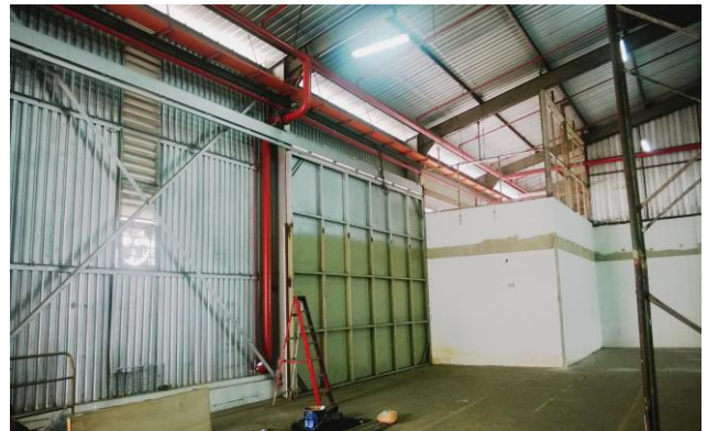
Warehouse entrance 2 internal view
