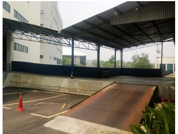
Loading area with 2 loading bays
