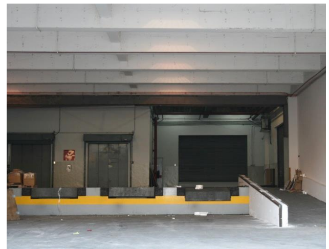
Loading area with 4 loading bays
